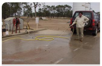
Washdown areas should be rinsed off after the vehicle has been cleaned, ready for the next vehicle
