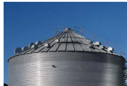
Silos with ventilation units
